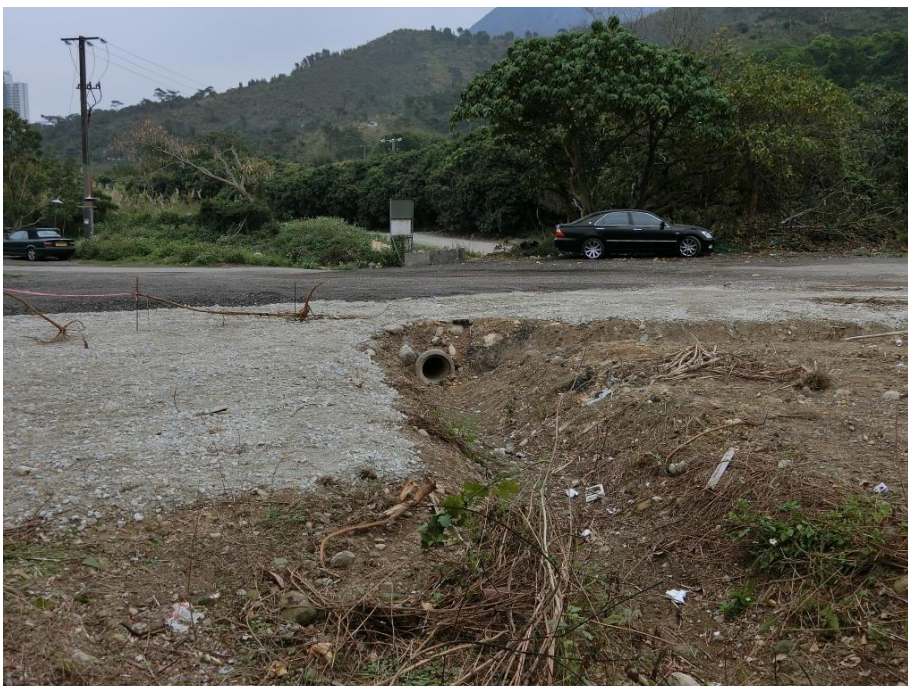
Photo 4 showing the end of underground pipe connecting to suspected illegal outfall 2 beside the illegal bridge (which is on the left of black private car in the photo) in Shek Lau Po
